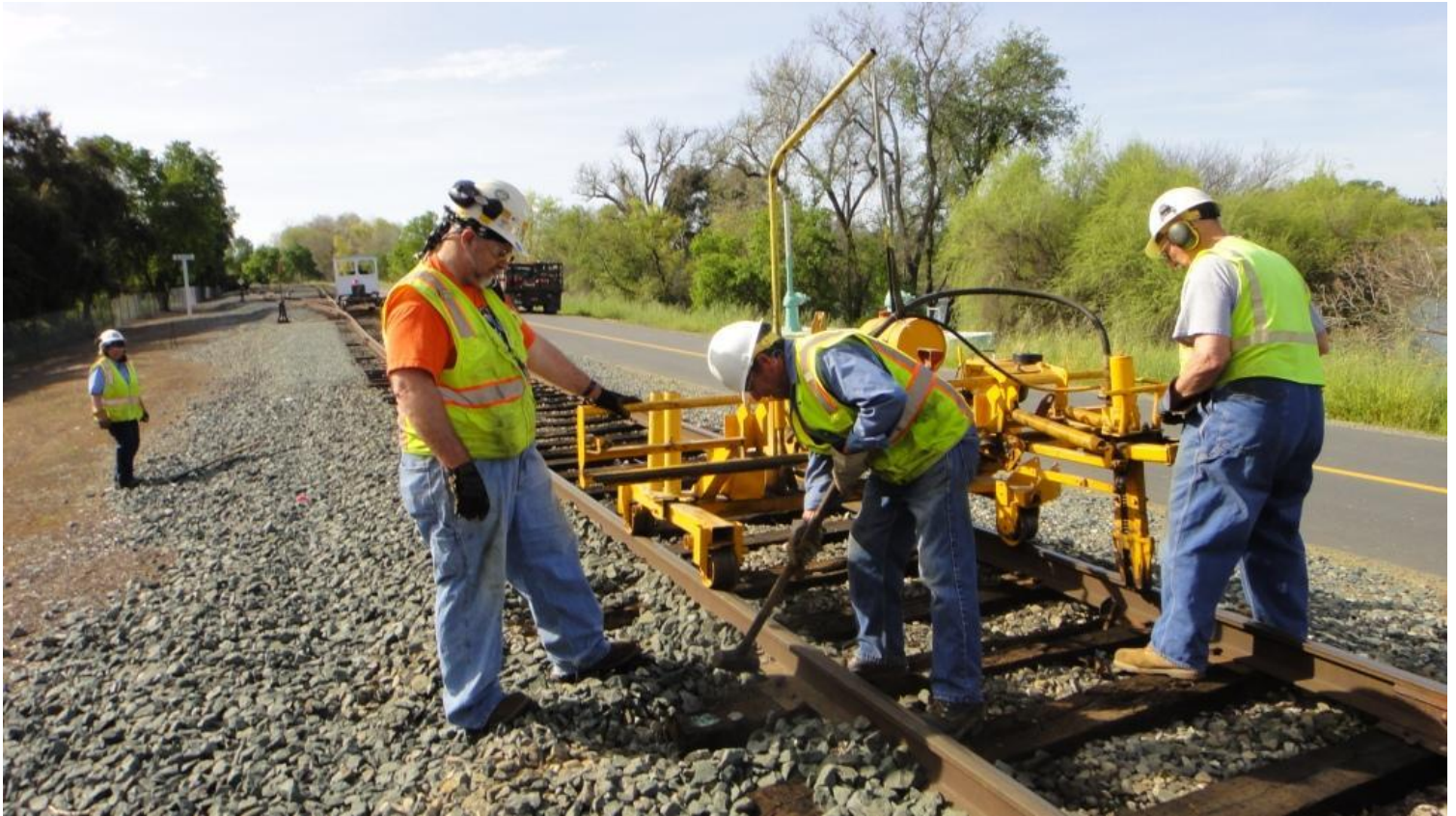
The spike-puller is deployed. Mike F. and Mike T. straighten a bent spike so that the machine can grab it while Clem pulls spikes on the opposite rail.
