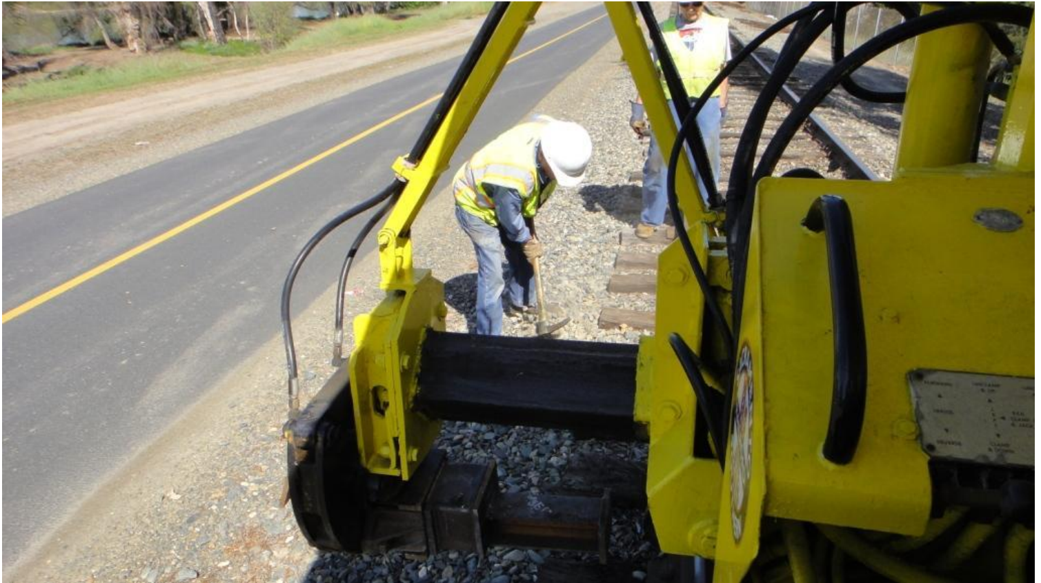
Mike T. removes rock from the ends of the ties so that the ram attachment can get low enough to shove the ties out. This is used when a tie disintegrates or breaks apart on the initial attempt to grab it.
