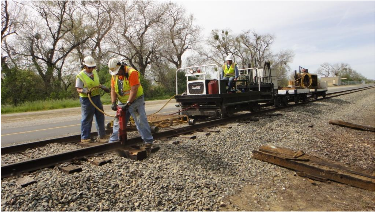
Clem guides the hose, Mike F., drives the spike, and engineer Mike T moves the whole operation along
