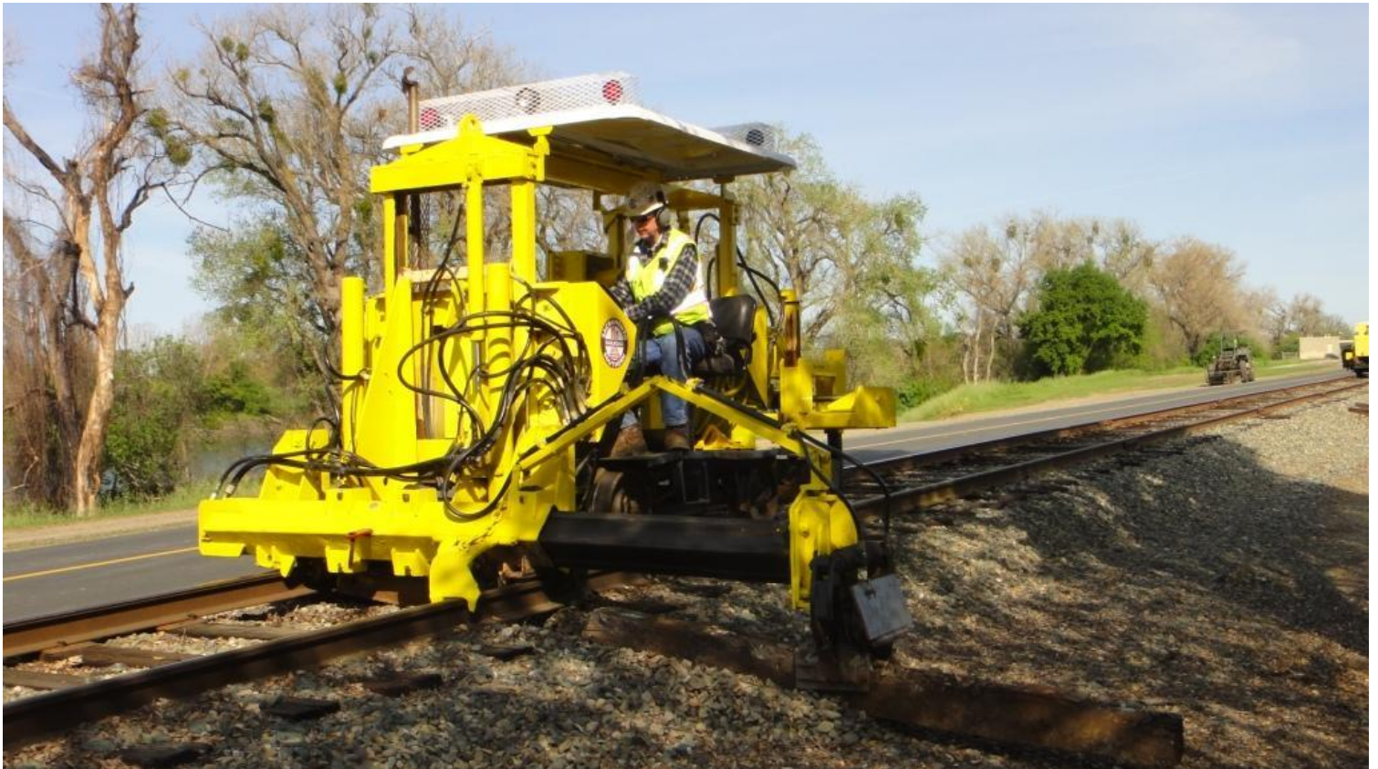
“Bring out your dead” – ties, that is... The Jackson 125 makes quick work of tie removal
