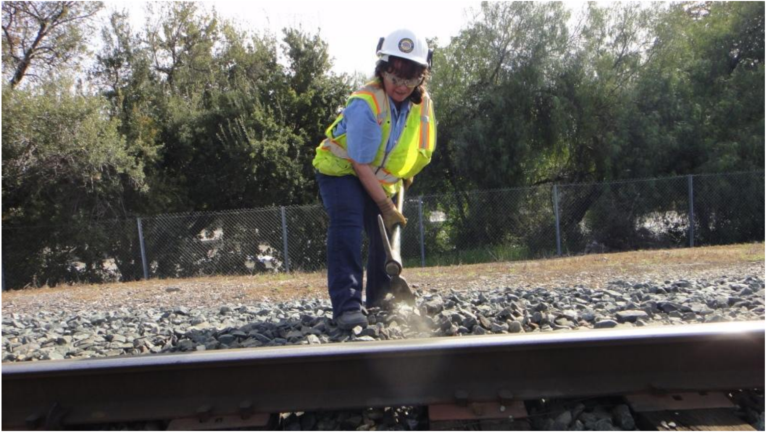
Pam digs out the ends of the ties to make it easier for the 125 to grab them.
